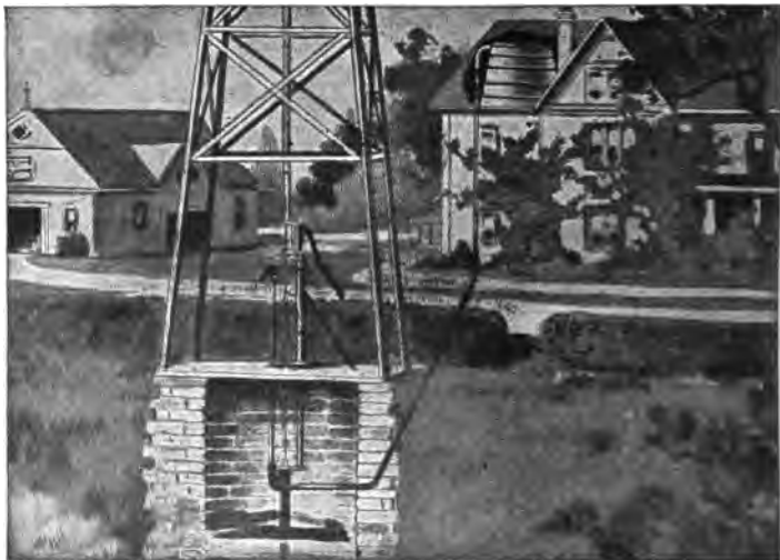
FIG. 186. — The windmill pumps water into the tank.
